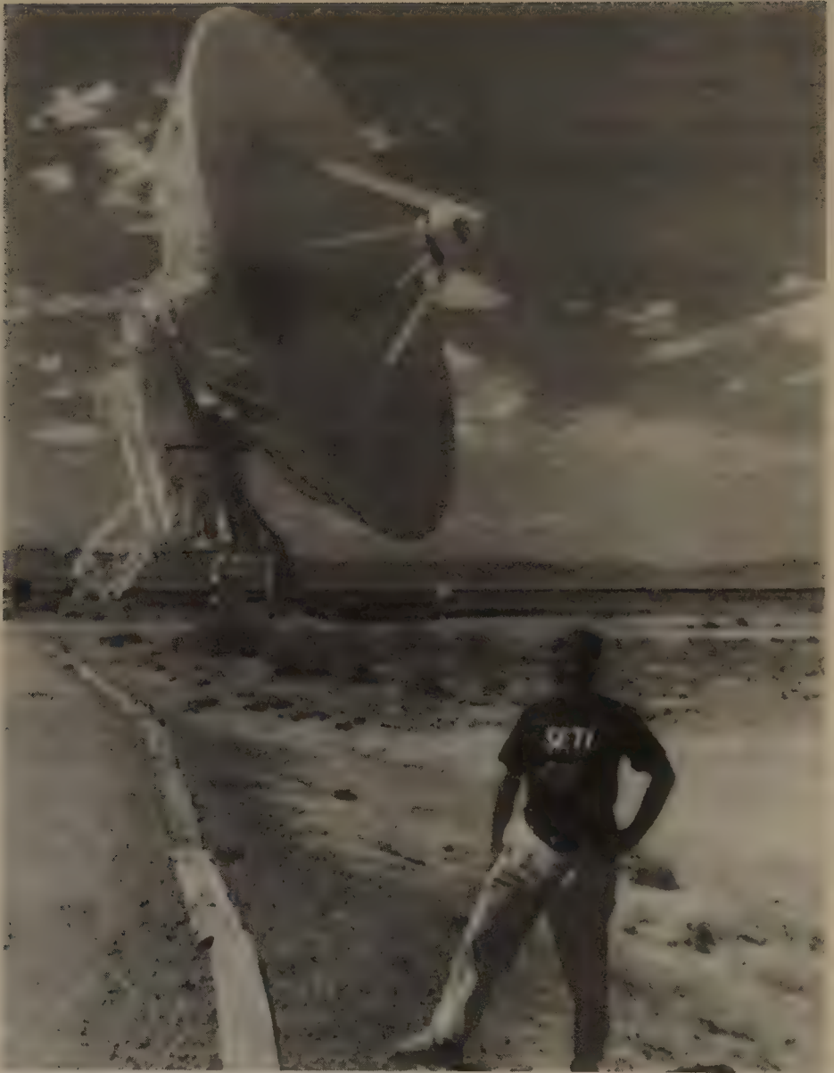
7.4 Dr. H. Paul Shuch poses in front of one of the antennas of the National Radio Astronomy Observatory's Very Large Array, Socorro, New Mexico. The VLA consists of 27 of these 82-foot-diameter (25 m) dishes, each weighing 230 tons. (SETI League photo, used by permission.)
