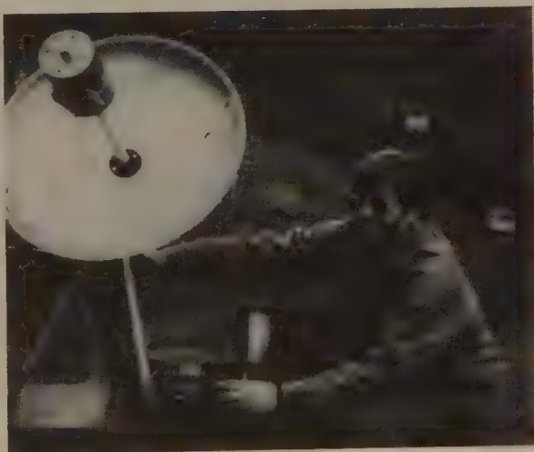
7.3 SETI League executive director Dr. H. Paul Shuch with a portable radio telescope. This system serves as a test bed for the hardware and software to be used for the Project Argus all-sky survey. The actual antennas used for SETI are much larger. (SETI League photo by Muriel Hykes, used by permission.)
